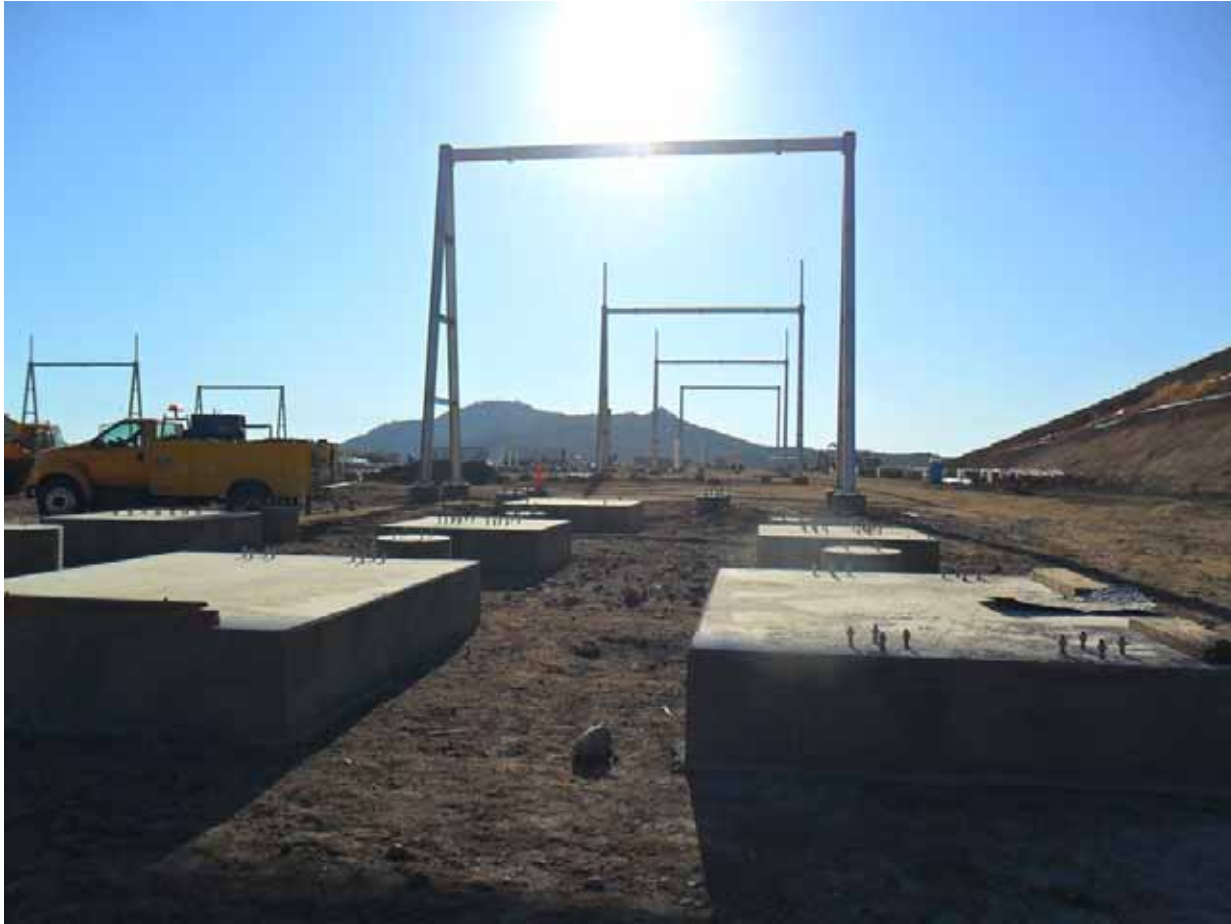
Steel erection at Suncrest Substation. Photo courtesy of Mark Meridith.
